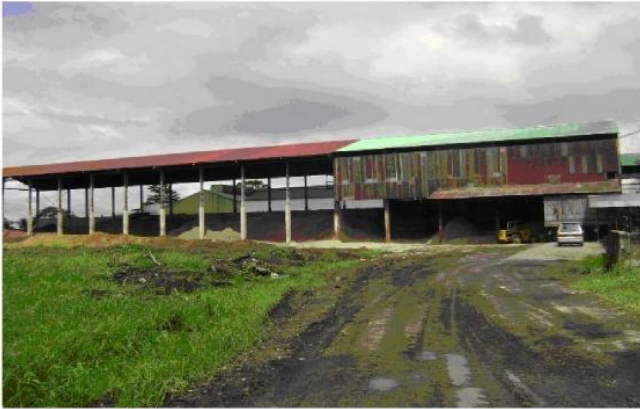
Figure 2.0: A sugar milling company in Leyte utilizes bagasse to fuel its boilers to generate steam used in its cane milling plant thus lowering energy costs for its operations [2].
