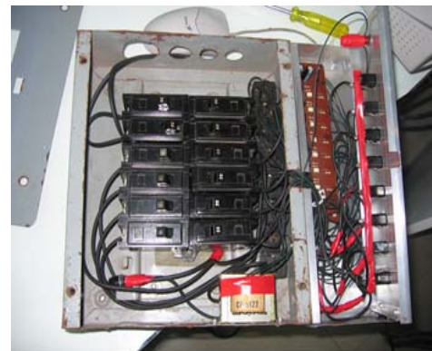
Figure 12 : The Panel Board Breaker and the Interface
