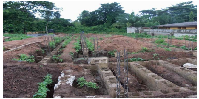
Permanent site of UNIFEMGA Nursery and Primary School under construction 5
