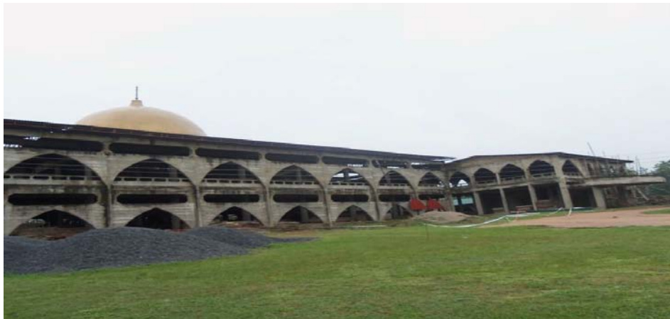
The new central Mosque under construction 3
