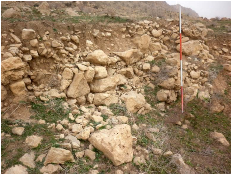
Figure 5 : view of one of the Terrace's wall of Part C
