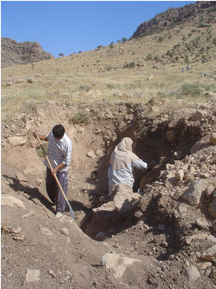
Figure 20 : View of dug pit in Part C
