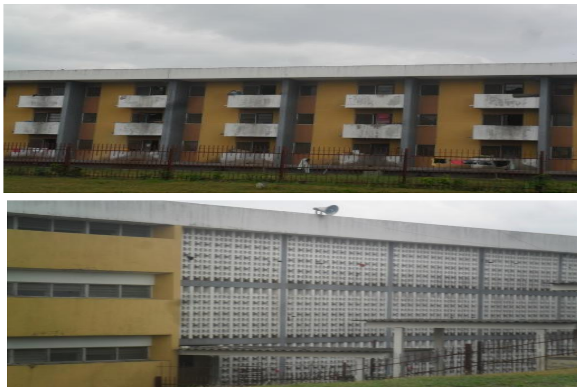
Figure 1 : General view of the case study building (a) roof overhang (b) screen wall
