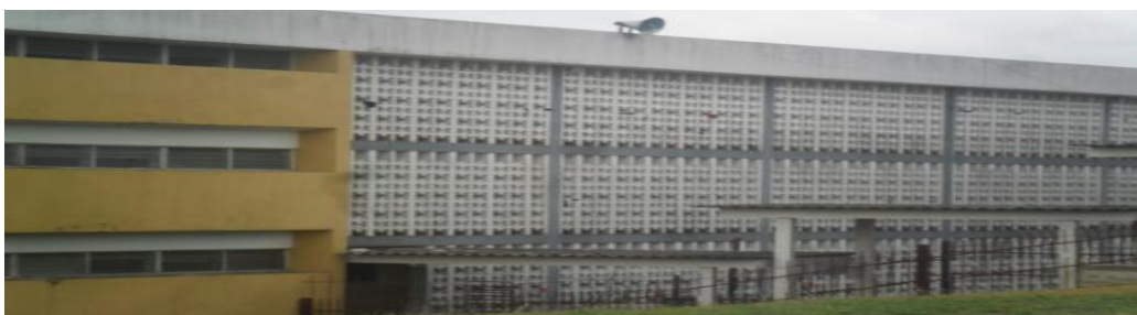
Figure 1: General view of the case study building (a) roof overhang (b) screen wall
