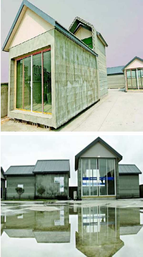
Figure 1 : Houses built by Shanghai WinSun Decoration Design Engineering Co., Ltd. within one day by using the technology of 3D printing (Photos: Liangfeng)
