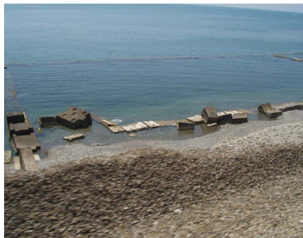
Fig. 25: Protection of the artificial shingle beach with using of the groin system and a long shore breakwater
