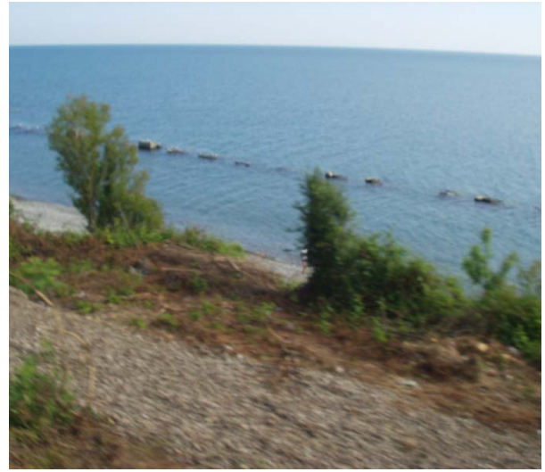
Fig. 14: Creation and protection of a beach with use of a faltering breakwater
