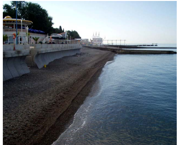
Fig. 21 : Protection of the artificial shingle beach with using of the groin system, wave-breaking wall of the quay and a long shore breakwater (beach of the 5*hotel "Black Sea")
