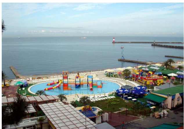
Fig. 28: Aqua-park, groin system in coastal and beach zones and moles of the port Sochi
