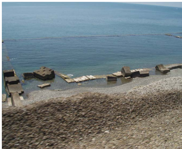
Fig. 24: Protection of the artificial shingle beach with using of the groin system and a long shore breakwater
