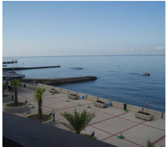
Fig. 20 : Protection of the artificial shingle beach with using of the groin system, wave-breaking wall of the quay and a long shore breakwater (beach of the 5*hotel "Black Sea")
