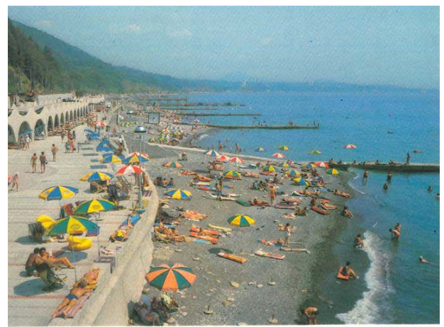
Fig. 16: Protection of the shingle beach with using of the groin system and wave-breaking wall of the quay
