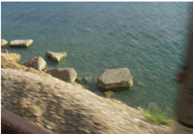
Fig. 5: The coastal site with landslide phenomena
