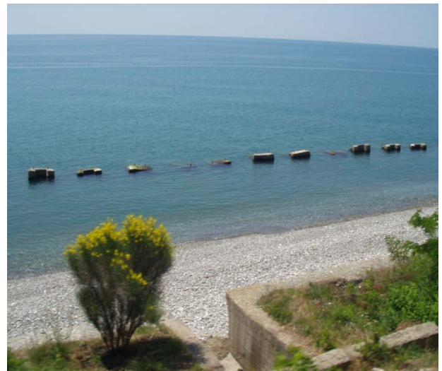
Fig. 15: Creation and protection of a beach with use of a faltering breakwater
