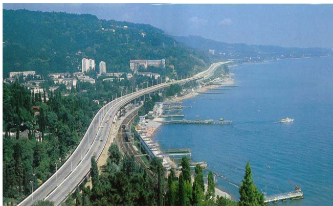
Fig. 3 : The railway and highway driving alongshore with groin system for beaches protection
