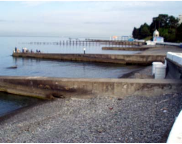
Fig. 17 : Protection of the shingle beach with using of the groin system and wave-breaking wall of the quay
