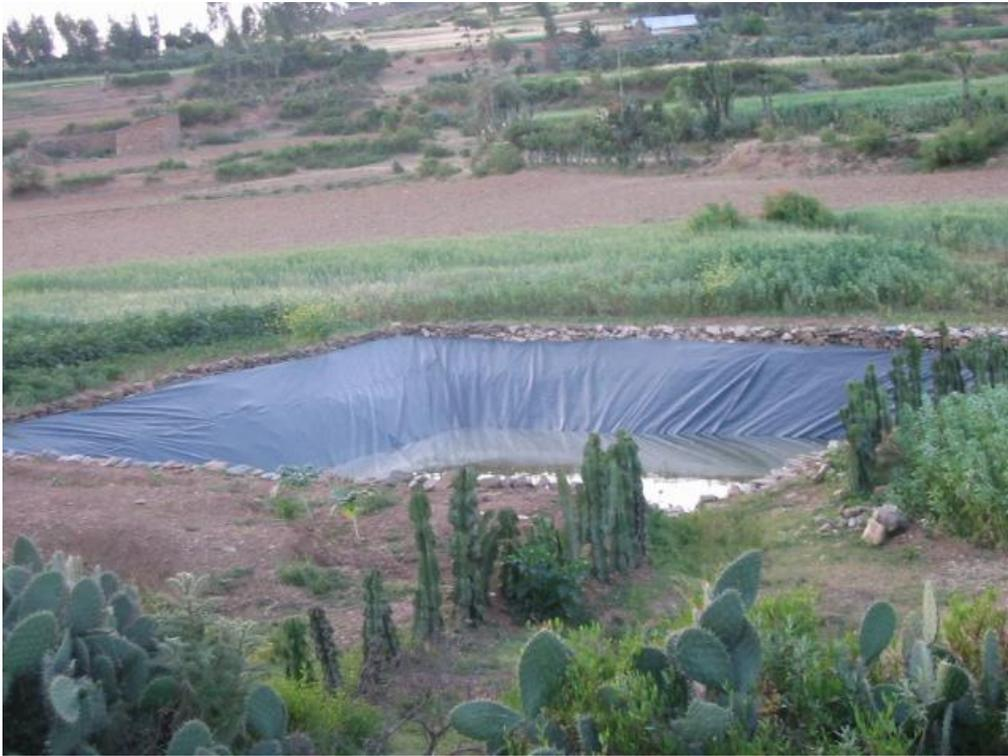
*Fig. 2 : Typical plastic lined pond in Tigray*
