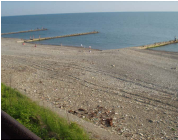
Fig. 18 : Protection of the shingle beach with using of the groin system
