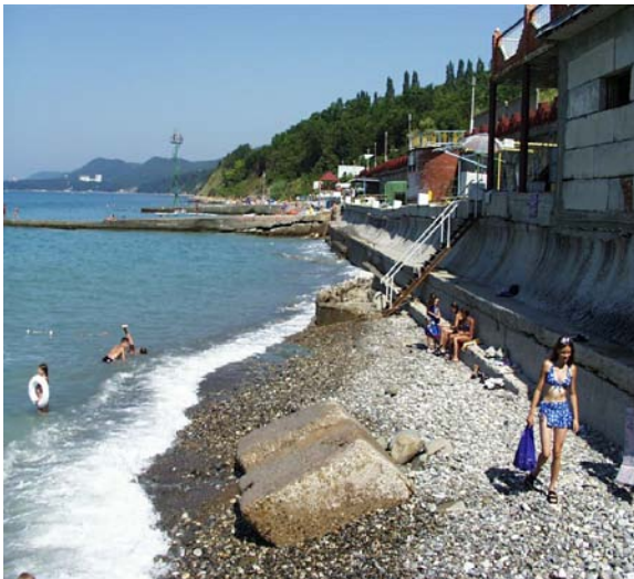
Fig. 12: Example of destruction of a wave protective wall. The beach near the wall is small
