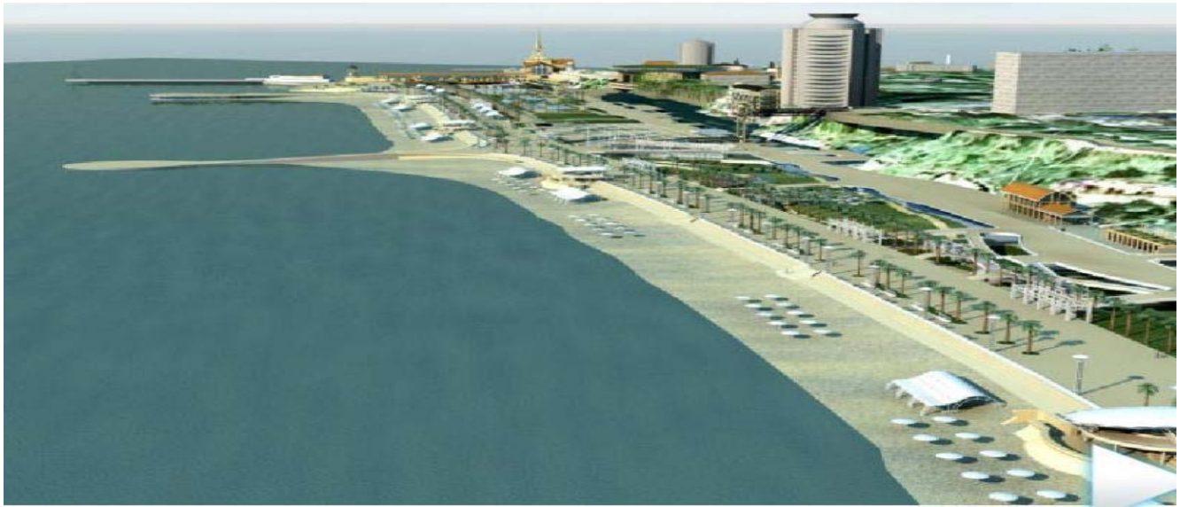
Fig. 31: The project on reconstruction of the main seaside embankment of Sochi with use of filtering underwater breakwaters of a macroporous design and the free pebble beach
