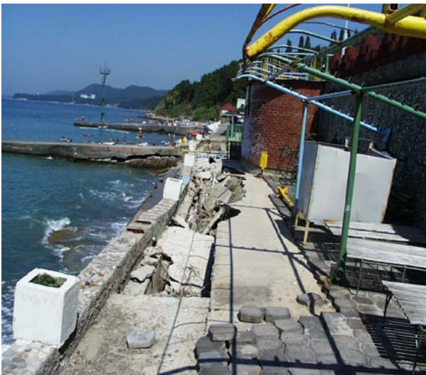
Fig. 11: Destroying of the wave-breaking wall from the marine and coastal party for want of a wave
