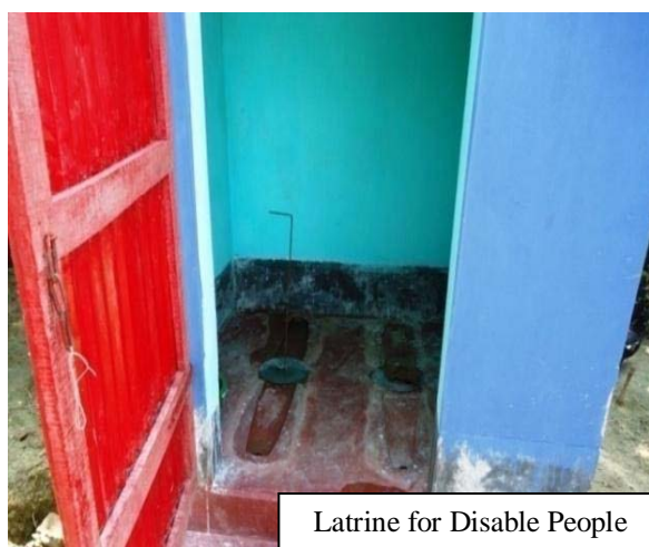
Figure 3: Installed pit latrines for vulnerable areas and people under PWASH project.
