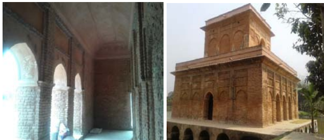
Fig. 3: Interior and outsider view of Hawakhana
