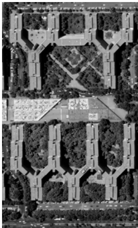
Figure 3: Blocks A 5 & B 4 and central market in Phase 1
