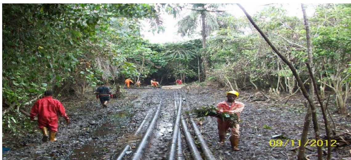
Figure 4: Right of Way Spill Clean up
