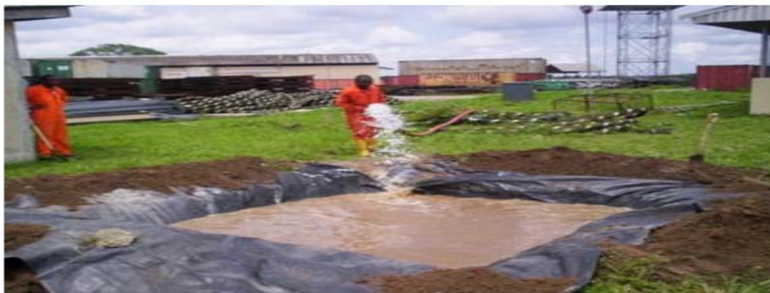
Figure 2: Lined Trench for Containment
