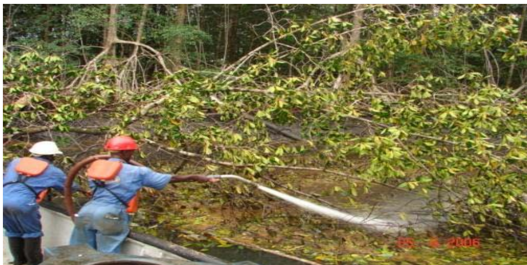
Figure 12: Low Pressure – High Volume Flushing of the Mangrove Ecosystem
