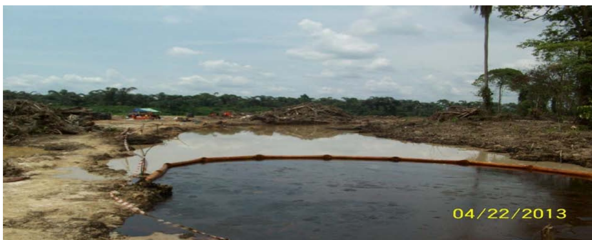
Figure 9: Oil Containment and Recovery in Progress
