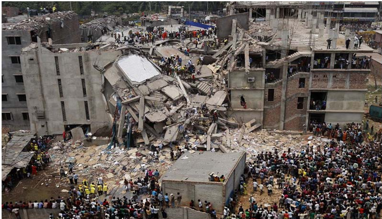
Figure 1 : The Rana Plaza collapsed due to the poor building codes and working area. Out dated labour laws, and a lack of awareness of labour rights among workers
