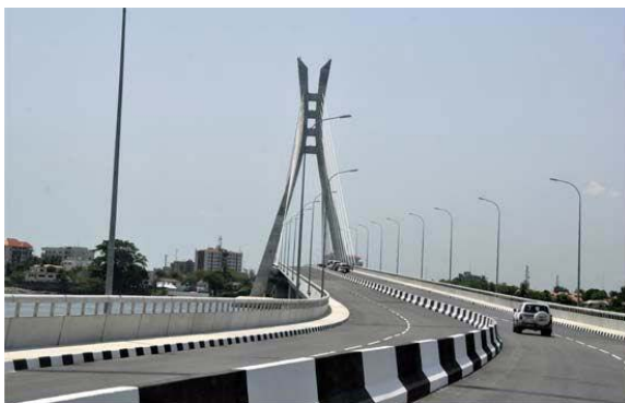
Fig. 1 : Lekki-Ikoyi Link Bridge
