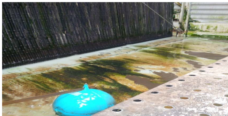
Photograph 1 : Visual inspection of the collecting basin - September 2014
