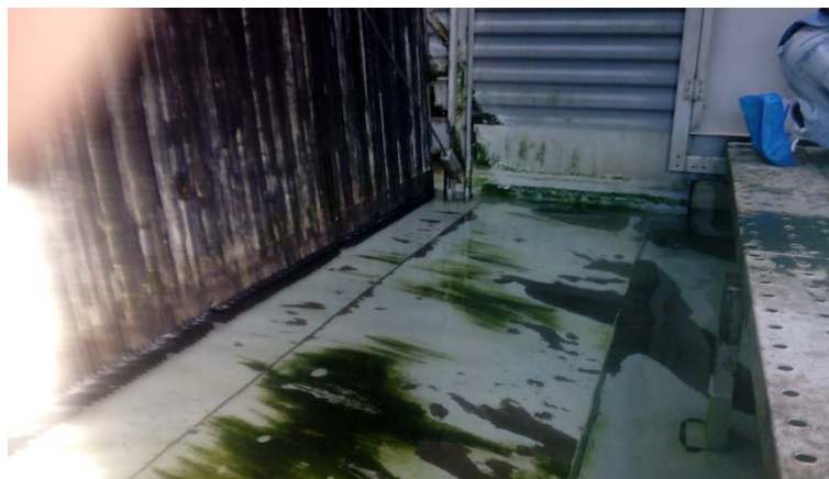
Photograph 2 : Visual inspection of the collecting basin - November 2014
