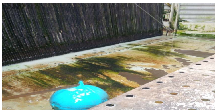
Photograph 1 : Visual inspection of the collecting basin - September 2014
