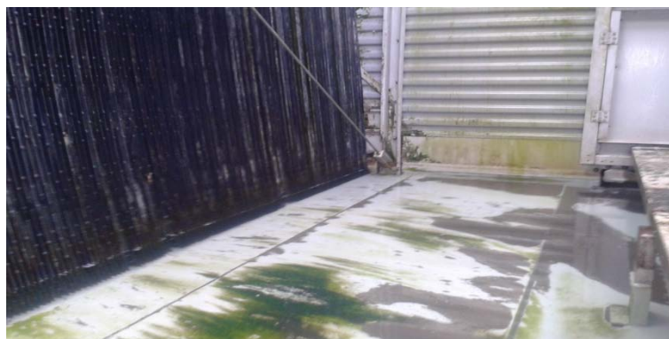
Photograph 3 : Visual inspection of the collecting basin - January 2015
