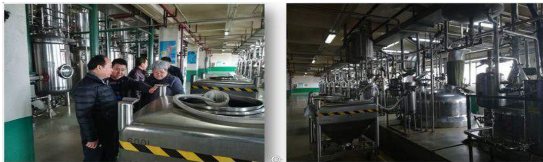
Figure 1: Factory Production Line of fermenting feed tank
