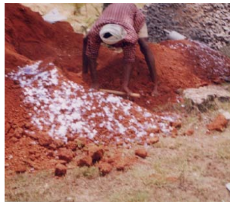
Fig.2(d) Mixing of Waste Plastics with Gravel
