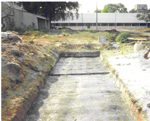
Fig. 2(c) Placing of Reinforcement Material in the Subbase Course
