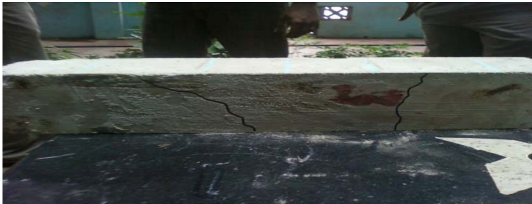
Flexure failure pattern of S.S.R.C beam
