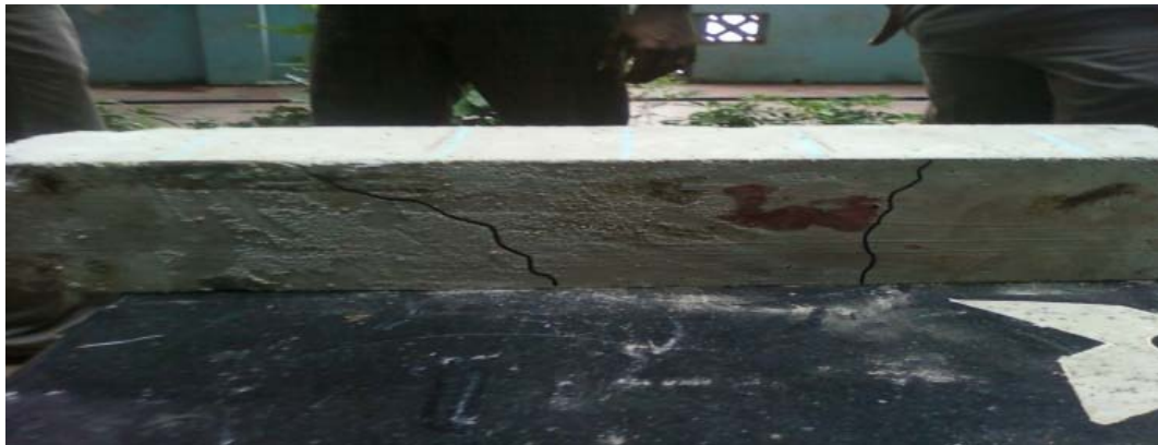
Flexure failure pattern of S.S.R.C beam
