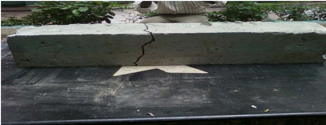
Shear failure of Plain S.S.C beam
