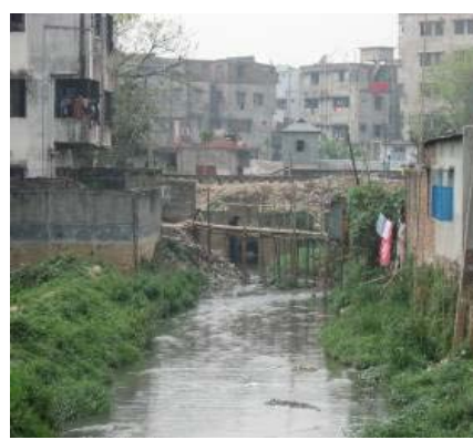
(f) Mohakhali khal (canal) near Mohakhali rail crossing
