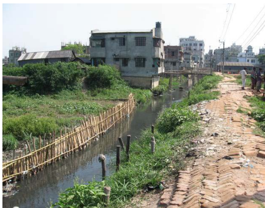
(c) End point of Shegunbagicha khal (canal) before the Kadamtala bridge
