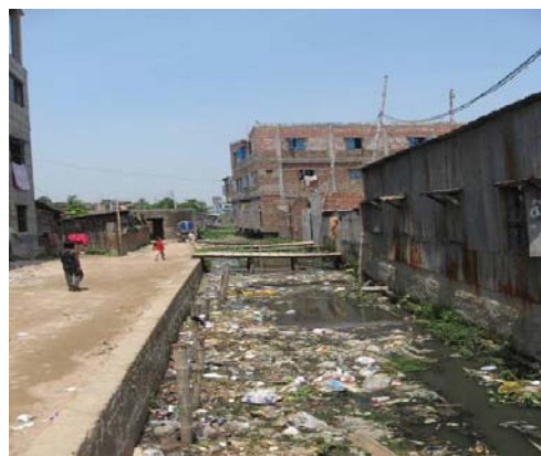
(b) Kayallanpur 'Ka' khal (canal) near Bosupara
