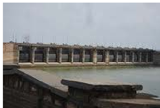
Fig. 2 : Mylavaram Reservoir Gates
