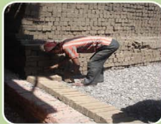
A layer of coal pieces is spread after two layers of bricks.
