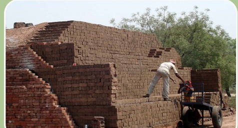
Brick pyramid is covered on the sides by faulty bricks or damaged bricks and sides are stuffed with coal.
