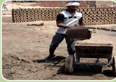
The mud is now carried in a trolley to the moulding area .
