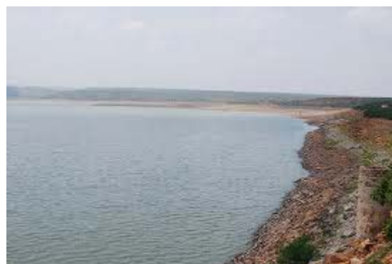
Fig. 1 : Mylavaram Reservoir North side
