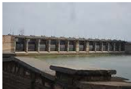
Fig. 2 : Mylavaram Reservoir Gates
