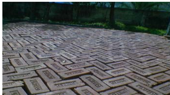
Figure 6 : Photograph of Close view - showing the interspaces 12.7mm in bricks
