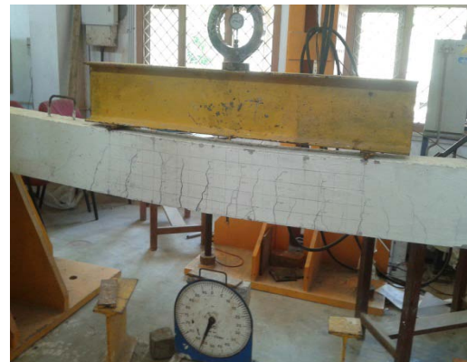
Figure 6 : Crack Pattern GPC-I Beam
