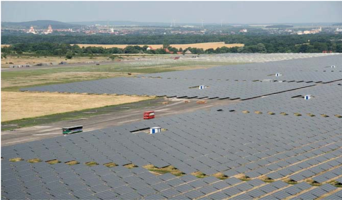
Figure 12 : First Solar 40-MW CdTe PV Array installed by JUWI Group in Waldpolenz, Germany, [19]
