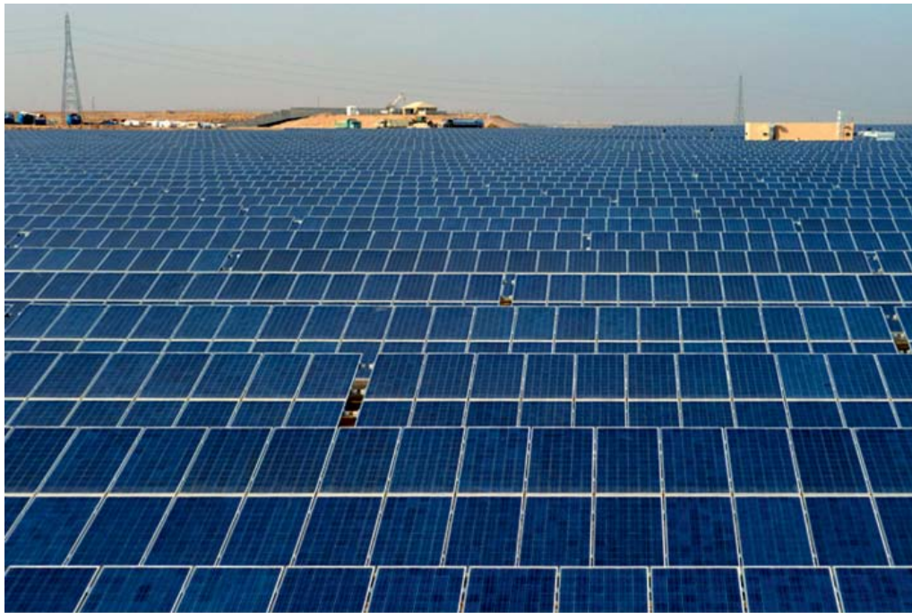
Figure 5 : Saudi Arabia: The ground-mounted photovoltaic plant with a peak output of 3.5 MW is located in Riyadh in the grounds of the KAPSARC (King Abdullah Petroleum Studies and Research Center), the largest oil research center in the world, Photo: Phoenix Solar AG, [4]
