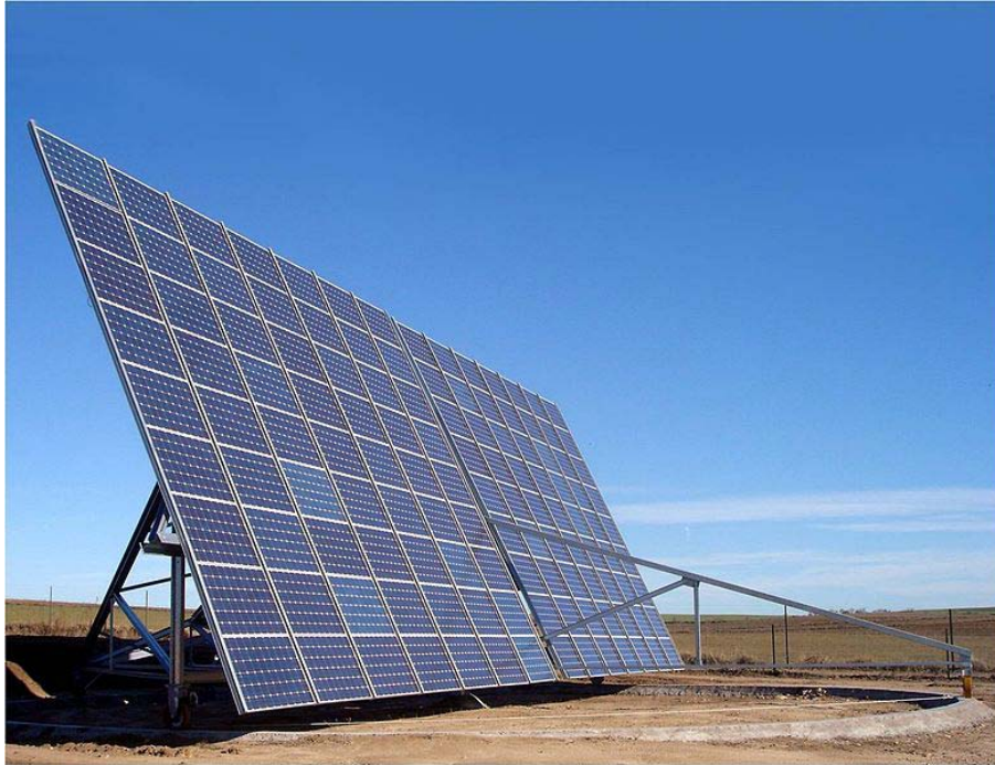
Figure 16 : Azimuth-altitude dual axis tracker - 2 axis solar tracker, Toledo, Spain
