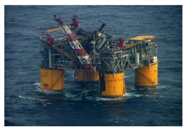
*Figure 3 :* Mars platform showing damage from Hurricane Katrina in 2005 (From http://en.wikipedia.org/wiki/Mars\_(oil\_platform))
