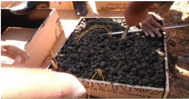
Figure 4 : Compaction of Concrete in Moulds
