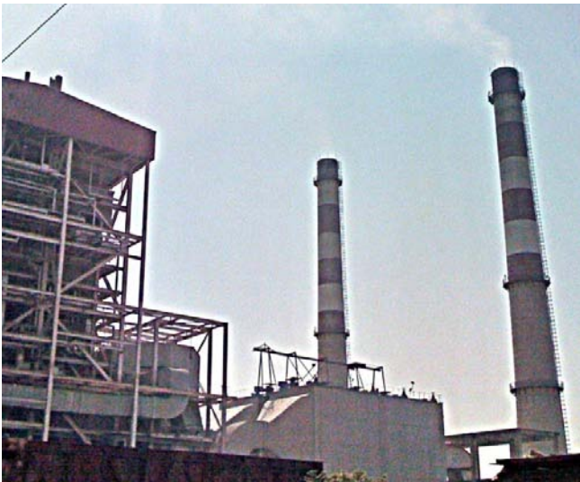
Figure 5 : Emission from the stack of Barapukuria thermal power plant
