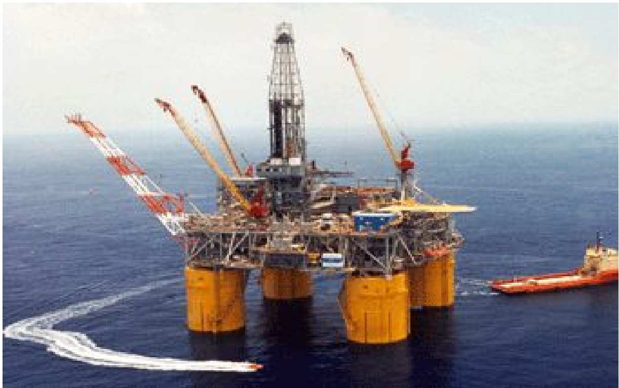
Figure 2 : Mars Tension-leg platform (From http://en.wikipedia.org/wiki/Mars_(oil_platform) )
