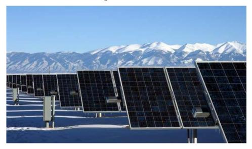
*Figure 14 :* Seasonally adjusted fixed-axis photovoltaic panels at the Sun Edison photovoltaic power plant near Alamosa, Colorado
