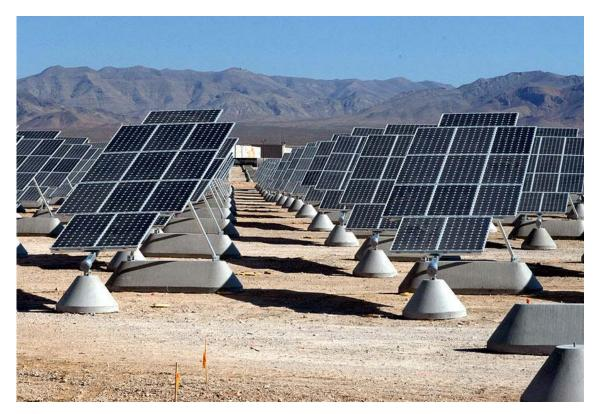
*Figure 17 :* Single axis trackers with roughly 20 degree tilt at Nellis Air Force Base in Nevada, USA. The arrays form part of the Nellis Solar Power Plant. Credit: U.S. Air Force photo by Senior Airman Larry E. Reid Jr,
