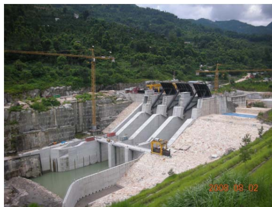
Fig.1 : MMHPP Dam view from Downstream
