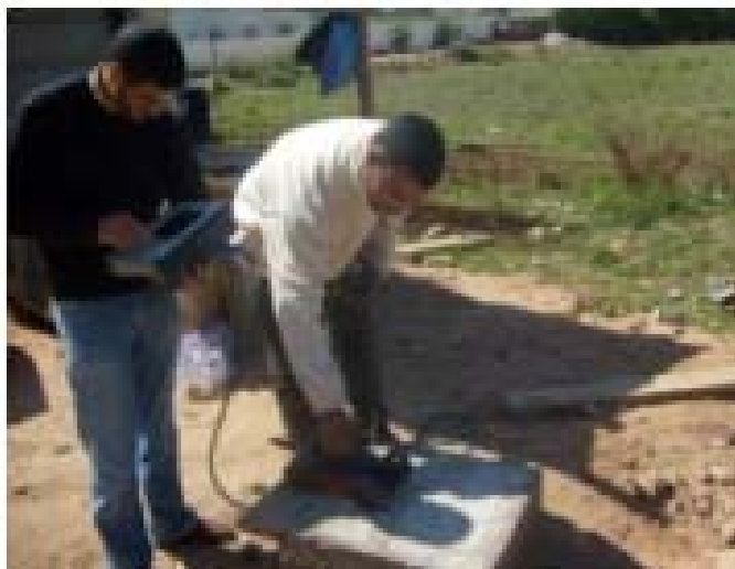
Figure 4 : Auscultation of reinforced concrete panels by GPR technology
