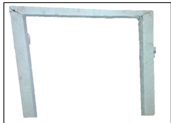
Figure 4b : Damage pattern for bare frame (M1) specimen
