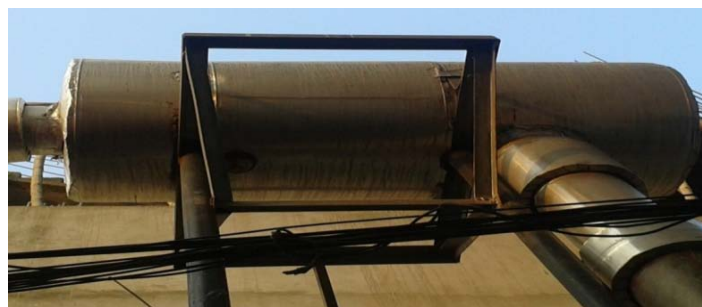
Figure 21 : After installation and at running.
