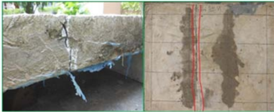
Figure 6 : Failure pattern of masonry slab using wire mesh
