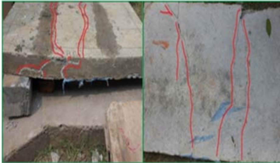
Figure 8 : Failure pattern of RCC slab using minimum reinforcement
