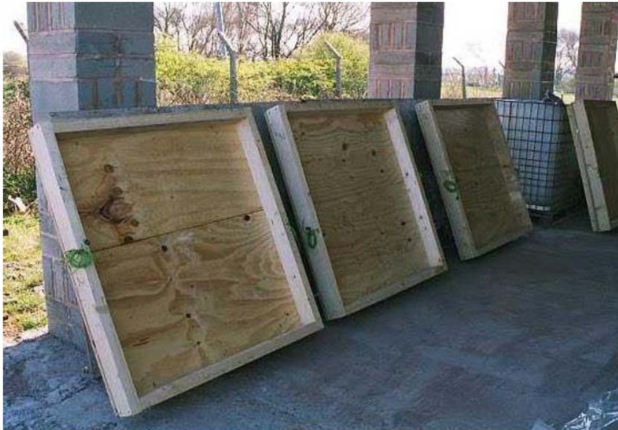
Figure 1: Wooden moulds for sprayed concrete panels
