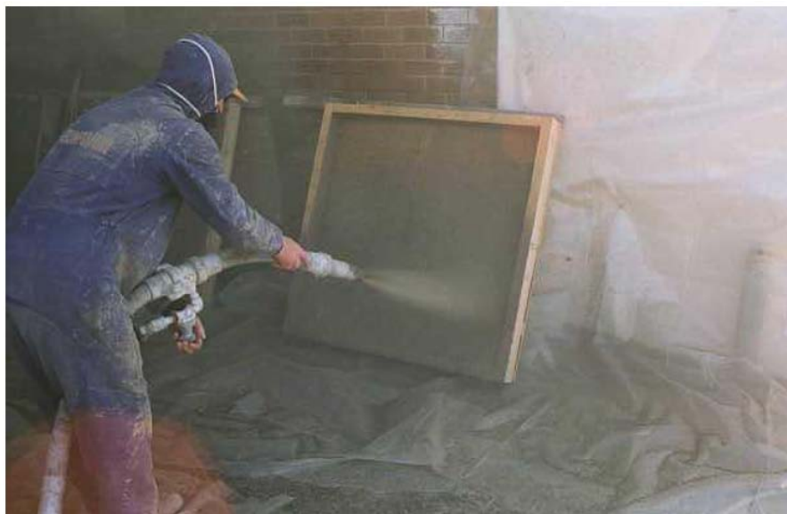
Figure 2: Production of sprayed concrete panels
