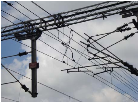
Fig. 3 : OHE Profile at Turn out Location
