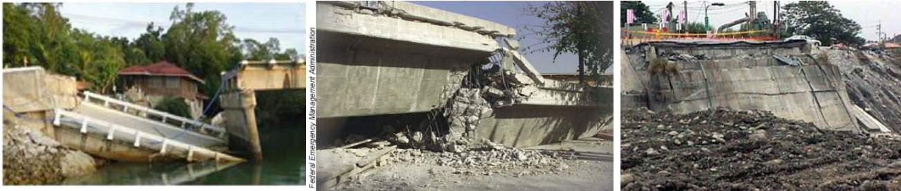
Figure 1 : Some failure modes of bridge abutment
