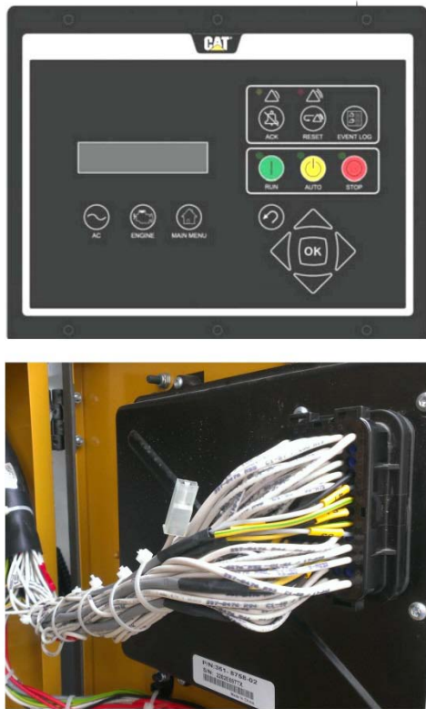
Fig. 3: Widely used DG controller, type EMCP 4
