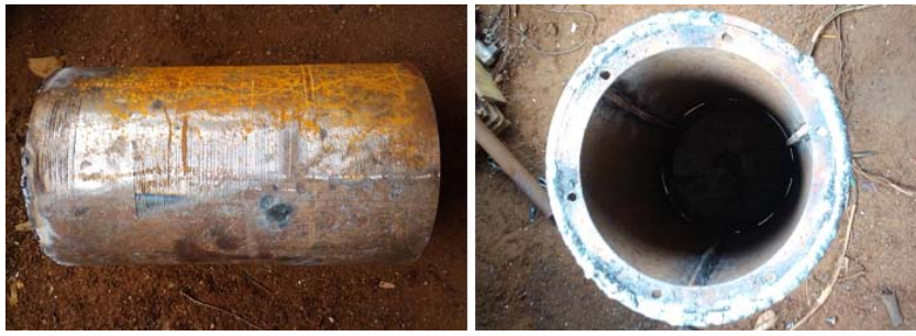
Fig. 4: The steel pipe cut to 375mm and the welded lifters
