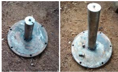
Fig. 6: Shafts welded to the round plates to make the flanges
