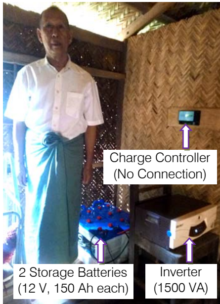
Fig. 10: The Villager and Components of his SHS
