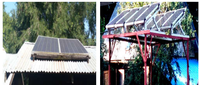
(a) Rooftop PV
