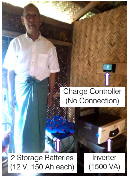
Fig. 10: The Villager and Components of his SHS
