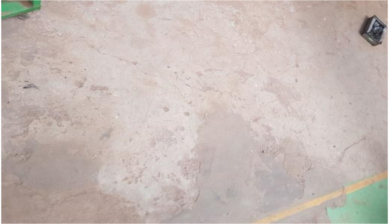
After - It is cleaned and overflow problem is solved.
