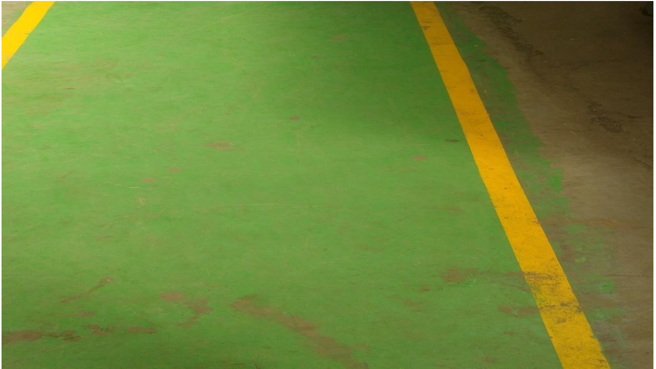
After - Patches are filled with Cement thus helping smooth material flow.
