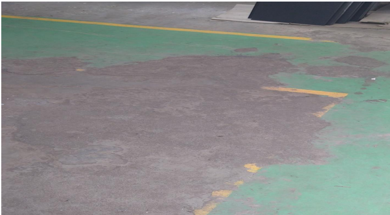
Before- Earlier patches on the floor were disturbing material movement using trolley.
