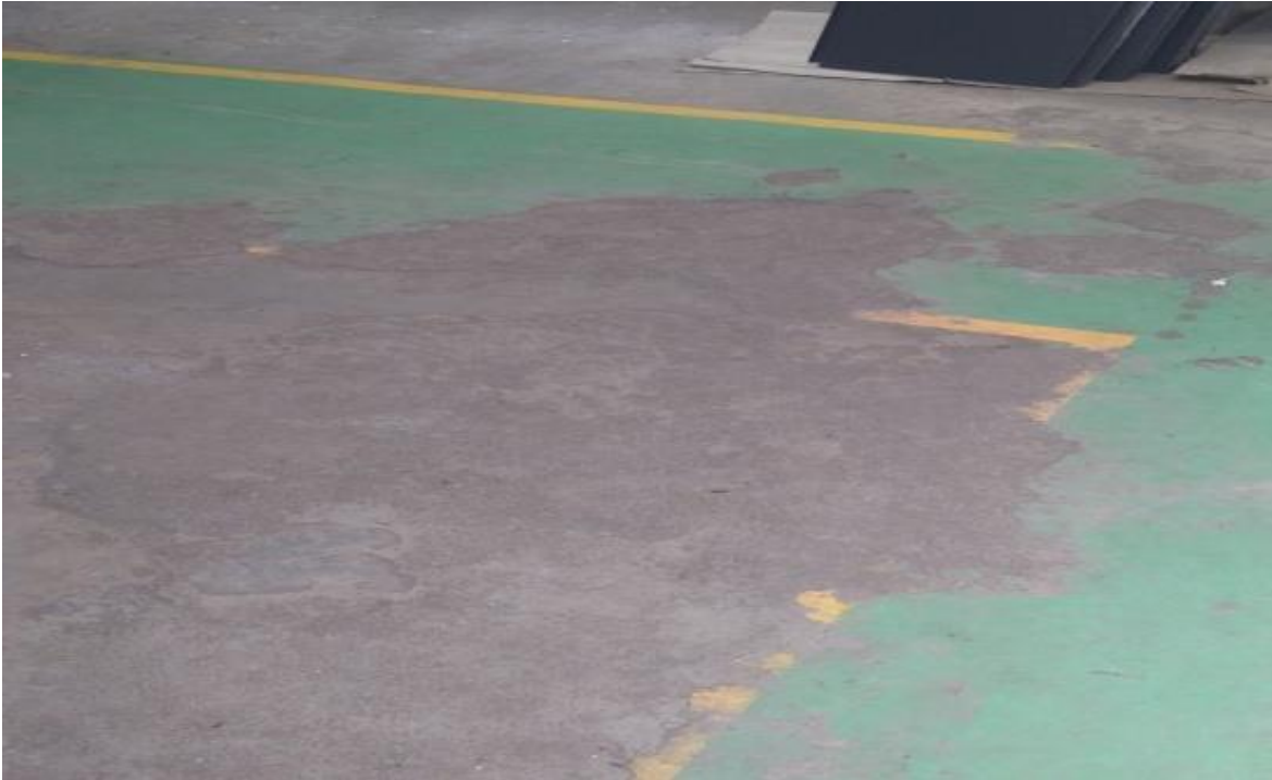
Earlier patches on the floor were disturbing material movement using trolley.
