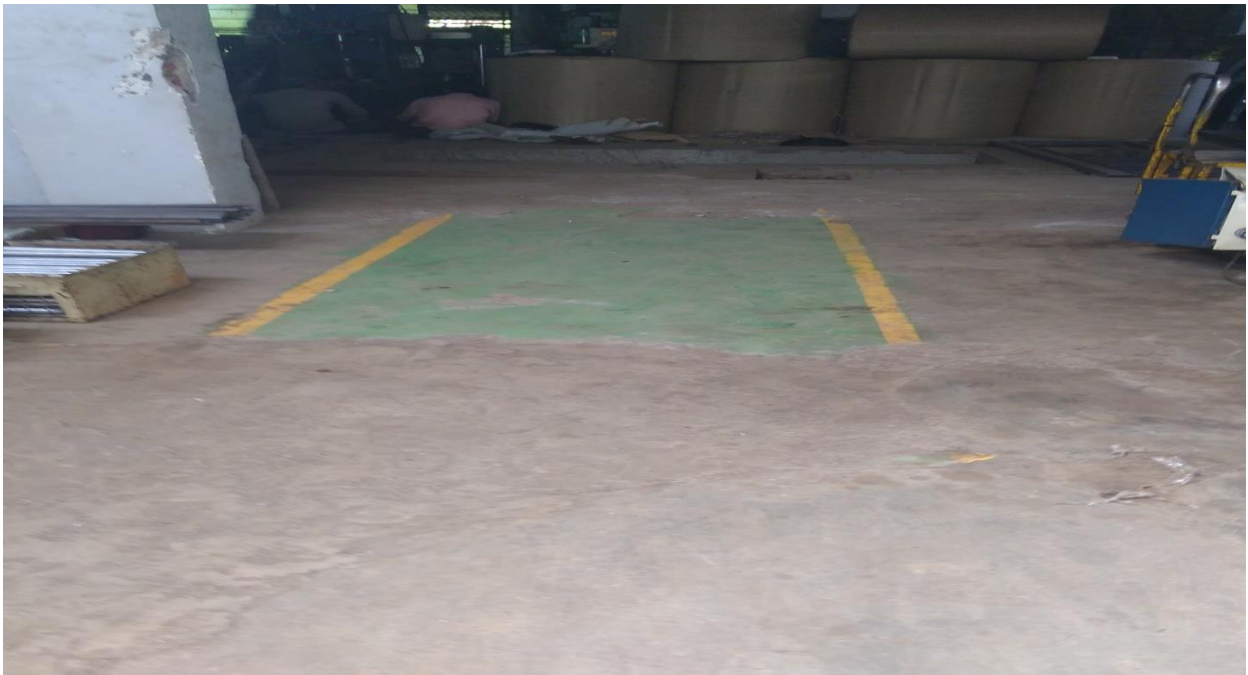
After - Tank is stored in central store room. The space is free for storing defective parts.
