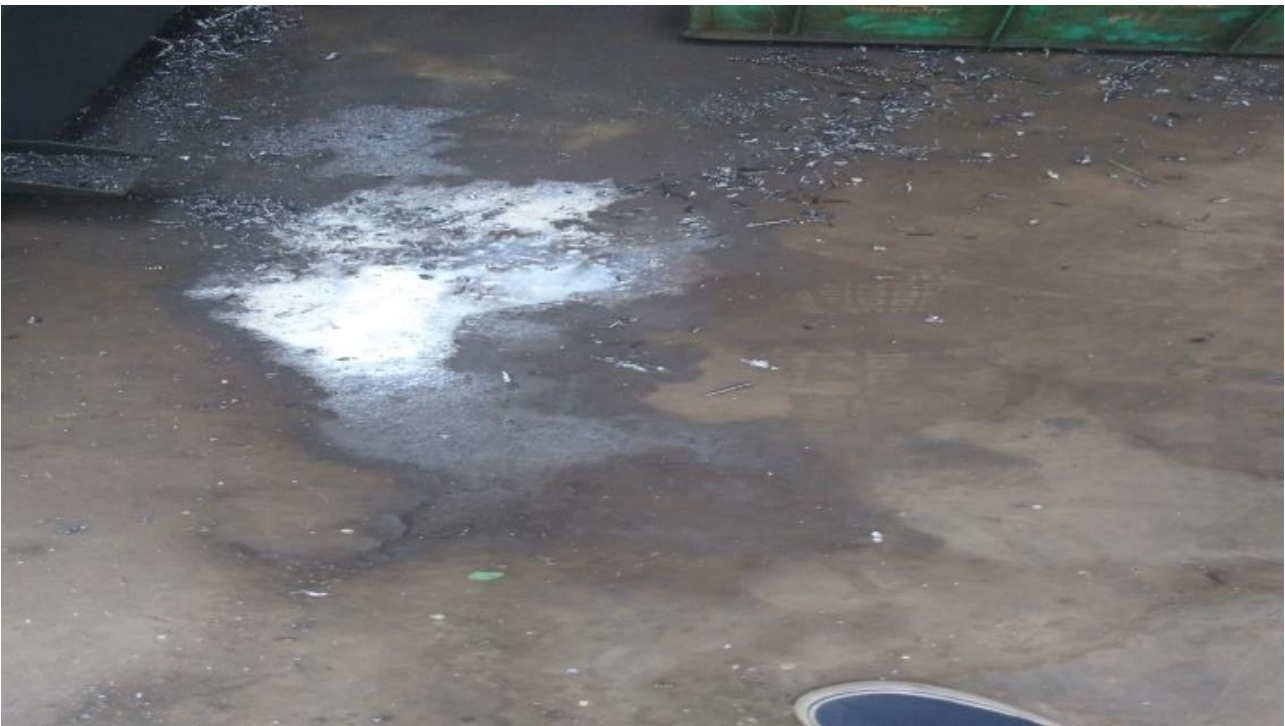
Before - Coolant overflows from the tank.
