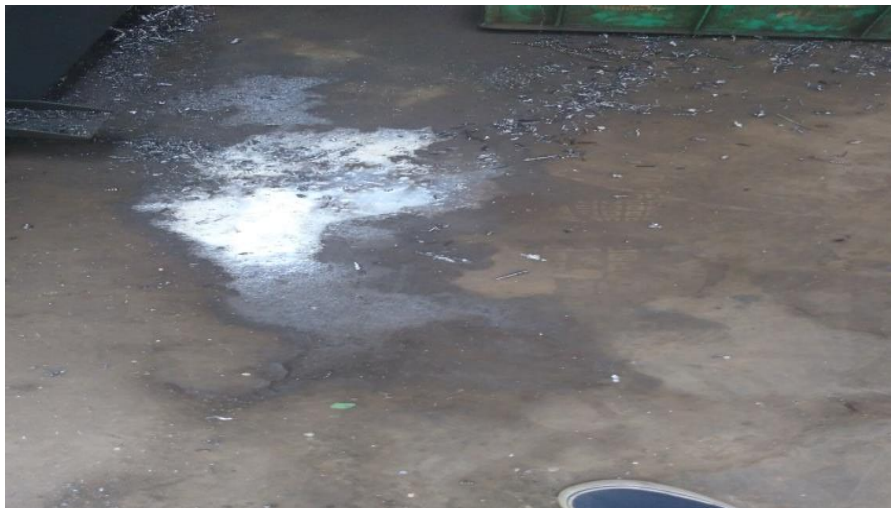
Fig. 1.6: Coolant leaked problem
