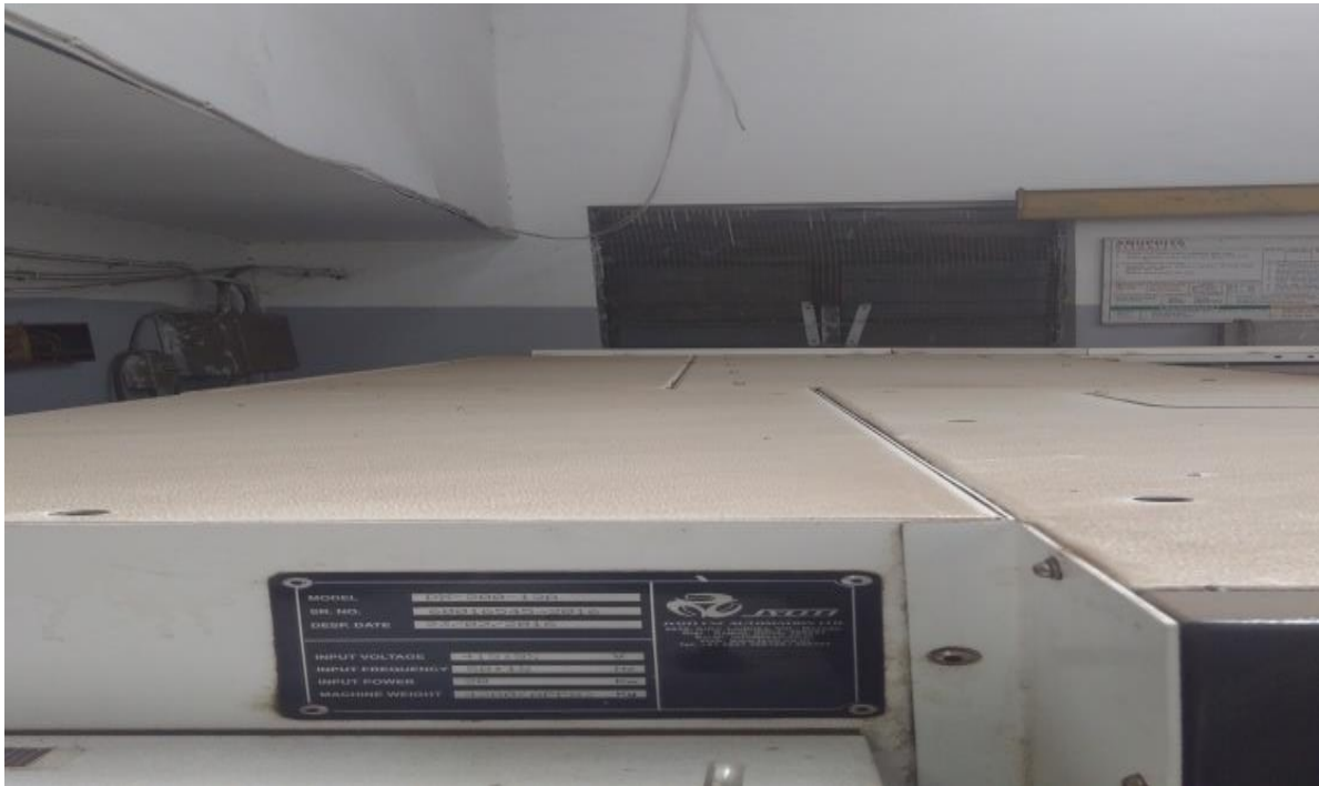
CNCs are not cleaned from top side.
