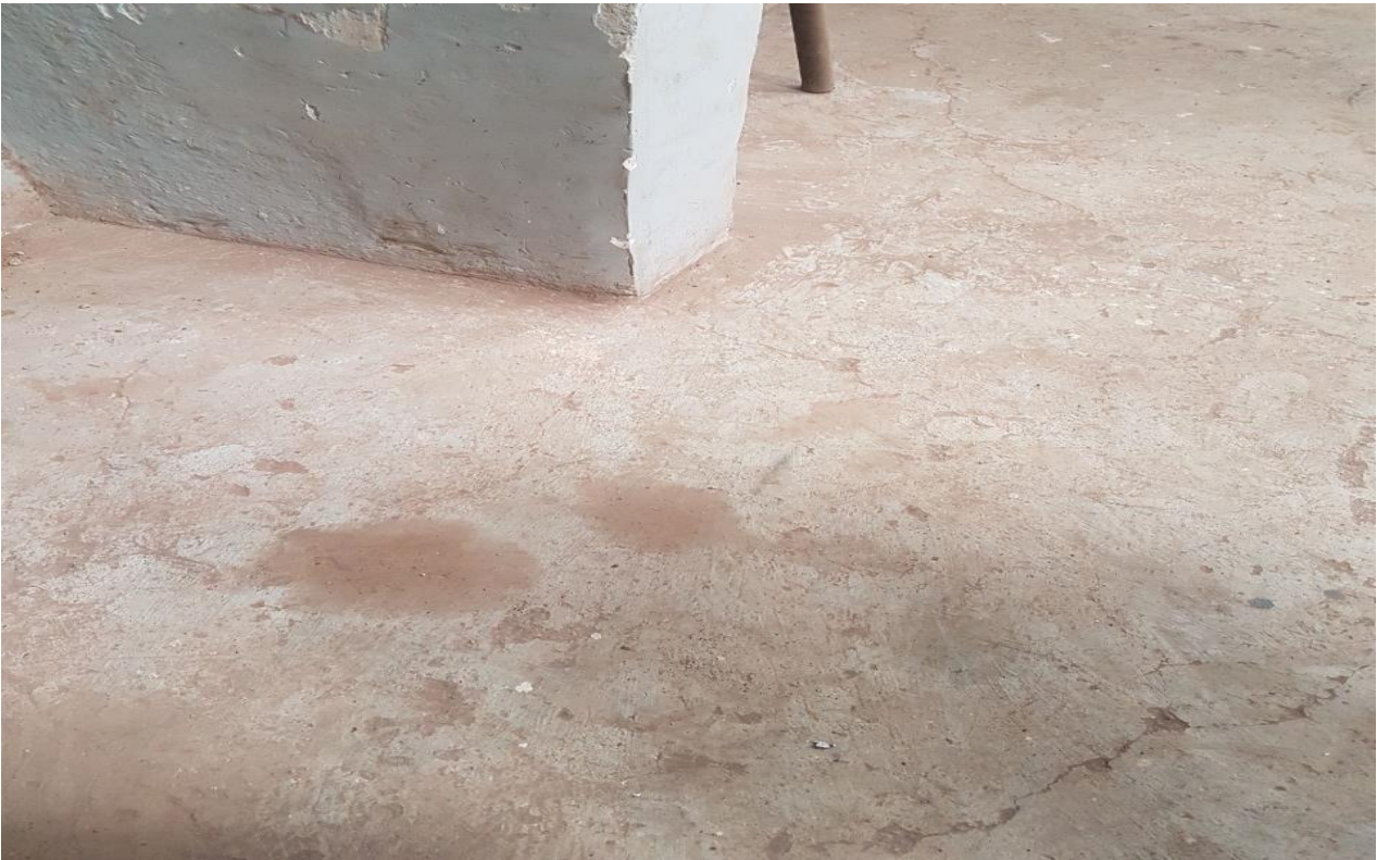
After - Space is dedicated for keeping trolleys whenever not needed.
