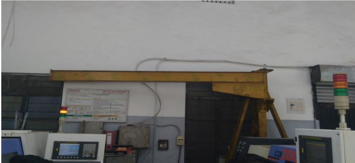
Crane used to load chuck for bell housing is still kept in between CNC machines even after its use is over.
