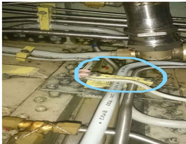
Figure 15: Pipelines Rubbing Against Each Other due to Zonal Vibration
