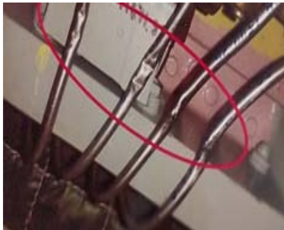
Figure 3: Damage to hydraulic pipelines followed by leakages and Pressure drop
