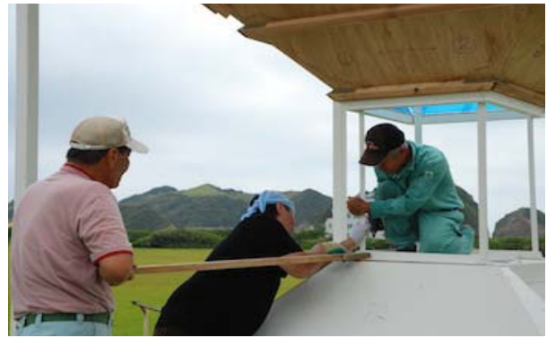
Fig. 6: A scene from the installing process (Tanegashima Space Center, 2014), photo: Yuri Tanaka
