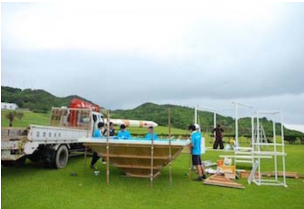
Fig. 5: A scene from the installing process (Tanegashima Space Center, 2014), photo: Yuri Tanaka
