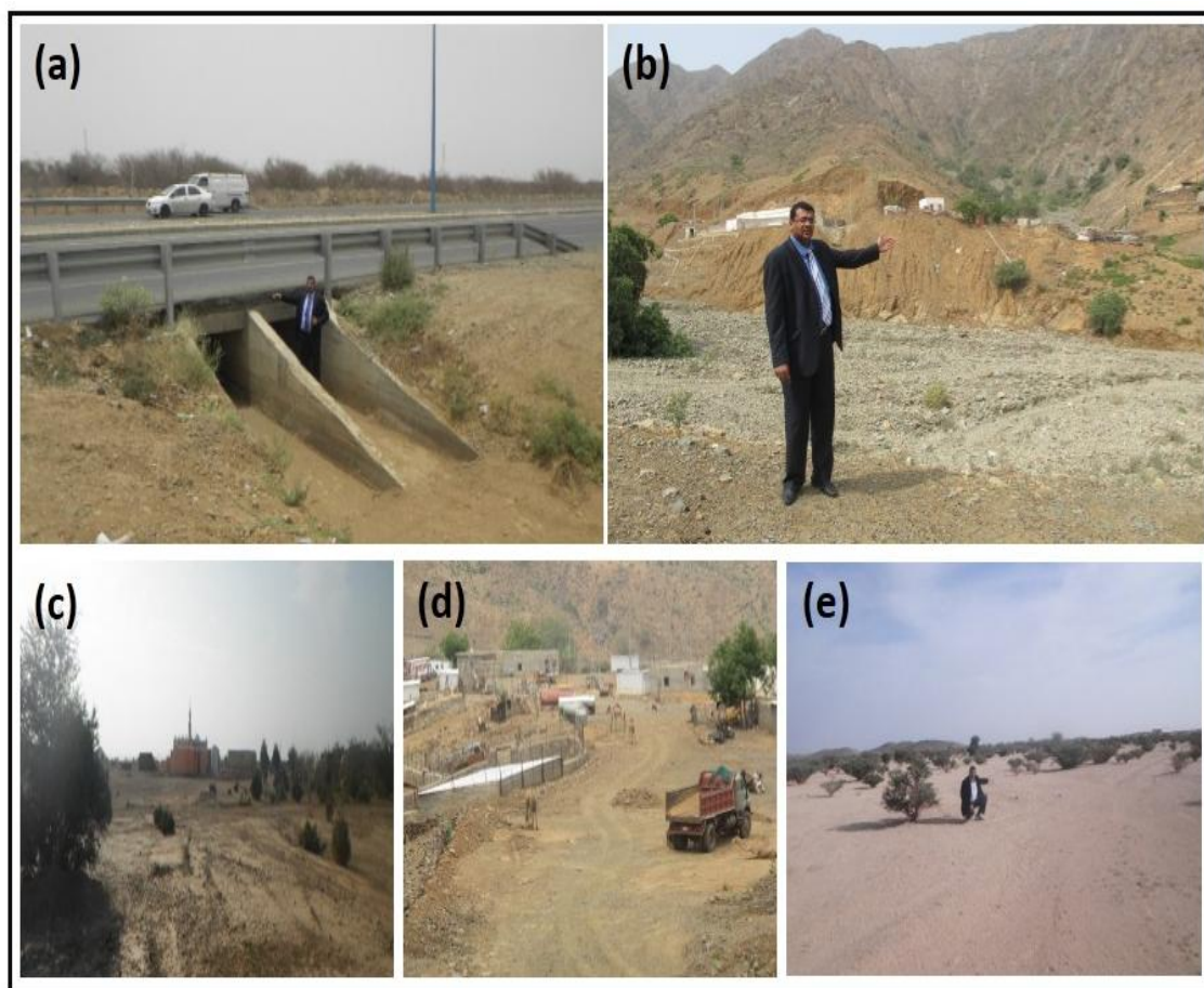
Figure 10: Field Study in the area of Study in 15/4/1440, (a) identify the characteristics of the existing structures below the Jazan-Abha road, (b) Urbanization in Wadi Bayad, (c, d, e) properties of Urbanization and valley down the road
