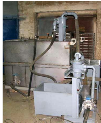
Figure 3: Water Treatment System.
