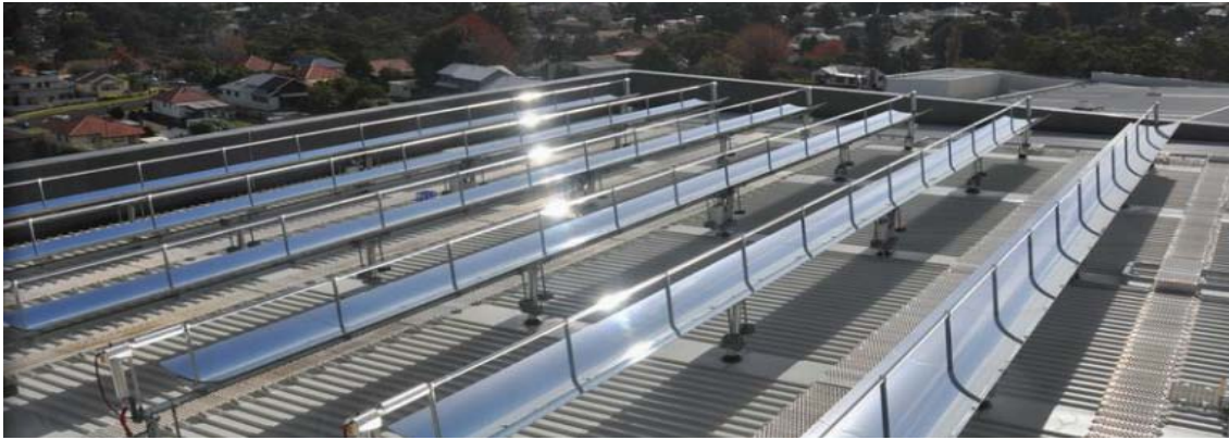
Fig. 1: Parabolic trough solar collector (PTC 1200)
